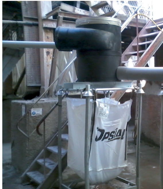
Cleaning of water coming from the manufacture of concrete blocks located in Clermond Ferrand, France
